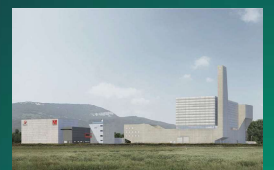
Future PHOS4LIFE® plant in Zuchwil, Switzerland
